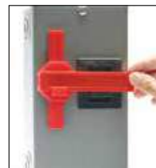
Slide Stop Bar into position over breaker
